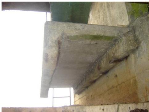
However, the catwalk extending perpendicular between the inside faces of the wingwalls had extensive areas of spalling concrete and exposed steel reinforcement (*shown on right below*).
