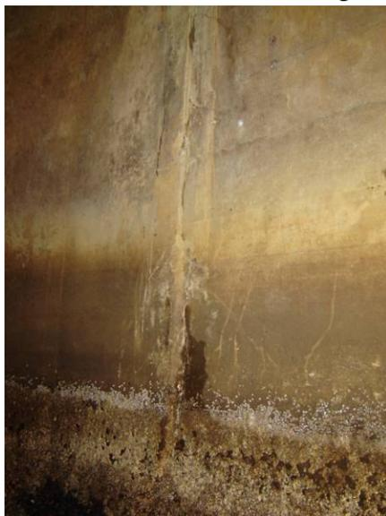
At this location, the patch material has lifted away from the wall. Similarly to the south wall, the vertical expansion joint has appeared to have opened up by approximately 3" at the bottom of the roof slab (*shown on right below*). However, unlike the south wall, the patch material filling the joint appears to be still bonded to the substrate (*shown on left*).
