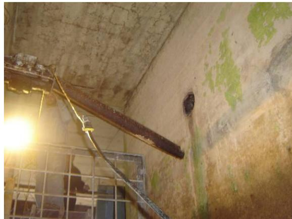
An abandoned, heavy rusted, 4" diameter steel conduit spans between the southerly and center walls, on the easterly side of the trash racks, approximately 12 feet above the invert slab and offset 3 feet west of the sewer line below. This conduit within the northern barrel of the sluiceway is broken and hanging from the center wall (*shown on right above*).
