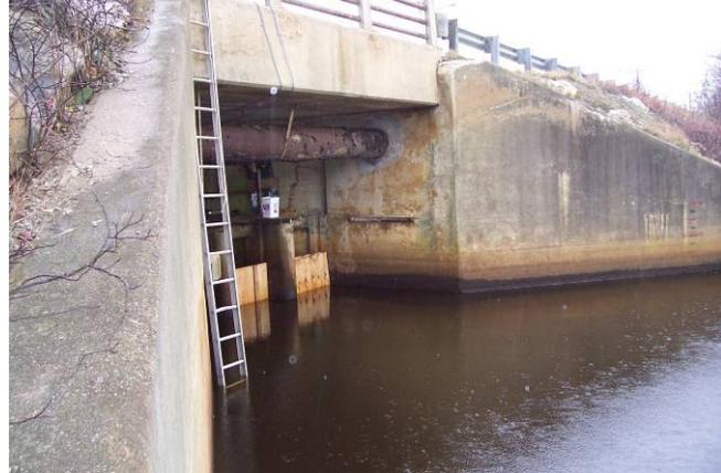
A 24" sewer line (*shown on left below*) spans between the northerly, center and southerly wall of the sluiceway, on the easterly side of the trash racks, and is located approximately 3 feet above the invert slab to the bottom of the sewer line.
