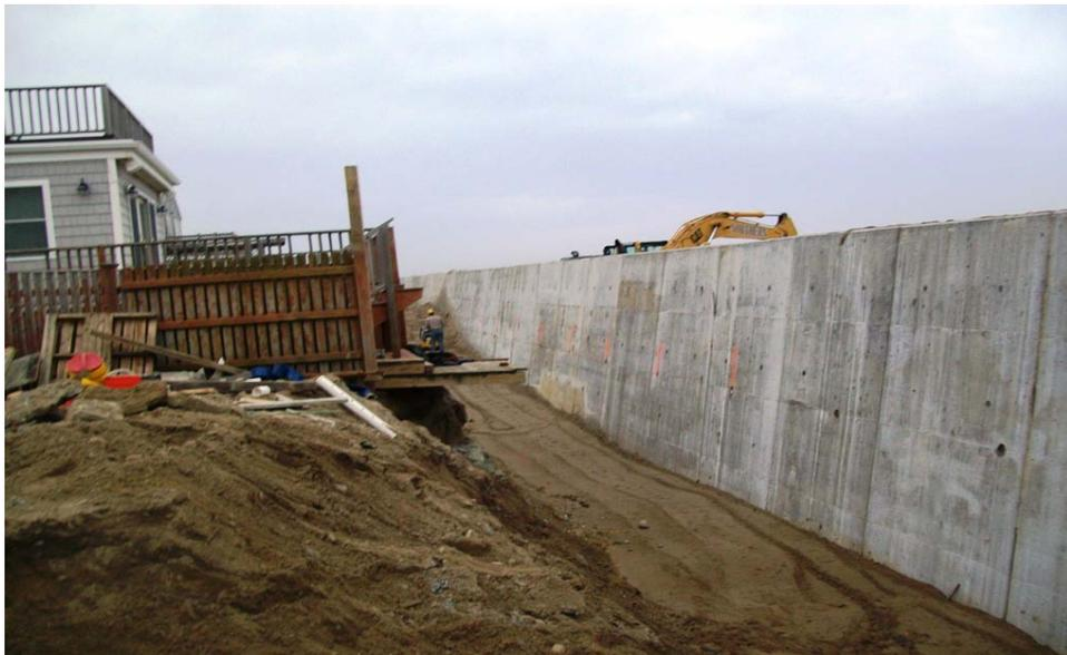
*Approximately 470' section of seawall running along Constellation to Farragut Roads failed in May 2010 after repeated fierce winter storms. The section was fully replaced by an emergency vote at special town meeting in August 2010.*
